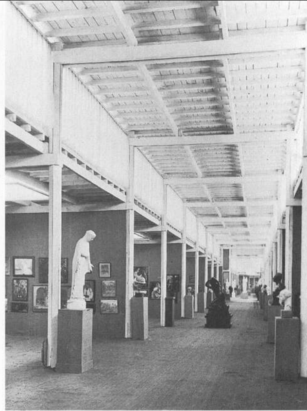
(above) Interior view of the Palais de Bois of the Salon des Tuileries, Paris, 1924. (right) Interior view showing the post and beam construction, Palais de Bois. (below) Plan and elevation, Palais de Bois.
